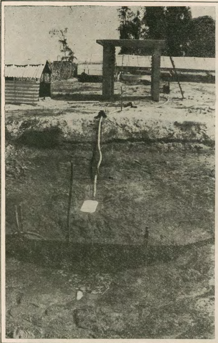
The sump of the hatchery for collecting filtered sea water, with the filter box exposed.
